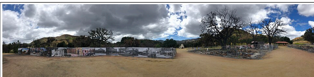
The Paramount Ranch following the Woolsey Fire and undergoing rebuilding in May 2019. The white church, central to Westworld season 1, remained standing.
